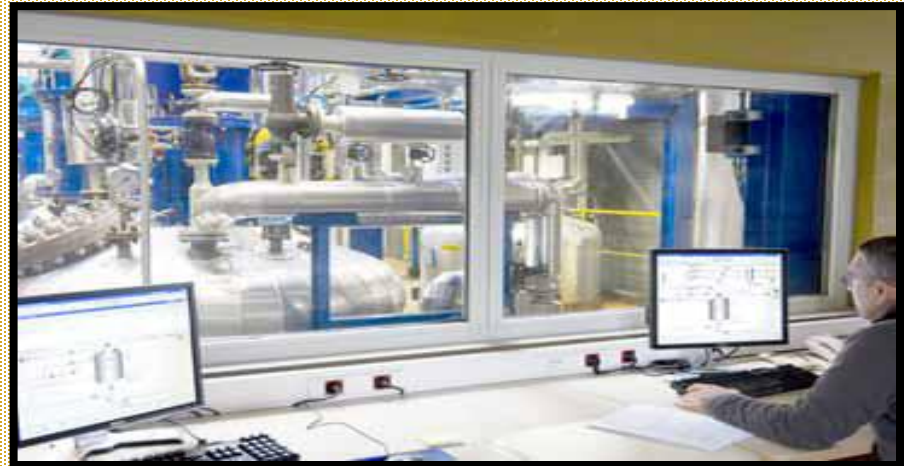
Control Room with Production Monitoring
